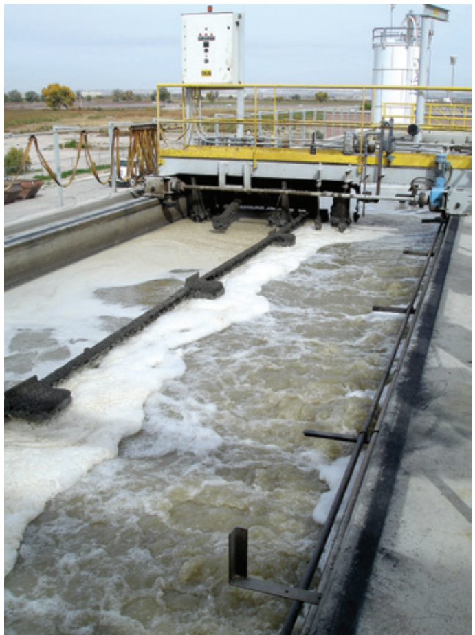
Wastewater Treatment Facility View
