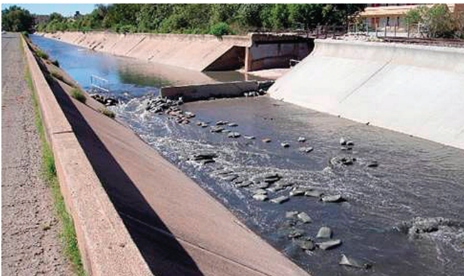
Raw sewage mixed with stormwater and treated with chlorine tablets flows past sandbags in the Nogales Wash used as a bypass for the dilapidated International Outfall Interceptor (IOI). The bypass of sewage into the Nogales Wash in Arizona was undertaken to facilitate repairs of the IOI at the border with Mexico. A dam designed to divert flows back into the IOI was breached by stormwater. Wastewater mixed with stormwater and flowed in an unlined channel as far north as the Santa Cruz River in Rio Rico, 8 miles north of this site (October 28, 2010).
