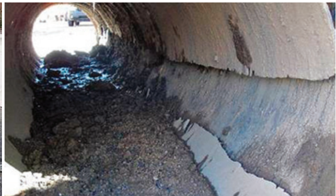
Damaged section of 24" diameter sewer pipe removed at the De Concini Port of Entry. The scour of the wastewater infrastructure in Arizona resulted from the introduction of sediment in Nogales, Sonora. This location is at manhole 1 in Arizona, immediately downstream of the border with Mexico (October 28, 2010).
